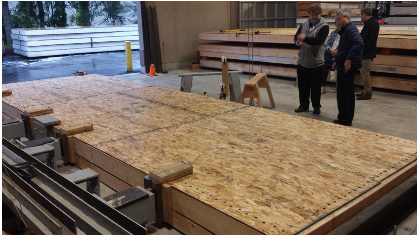
Figure 5. Test setup for a Part B SIP diaphragm connected to framing (before testing).
