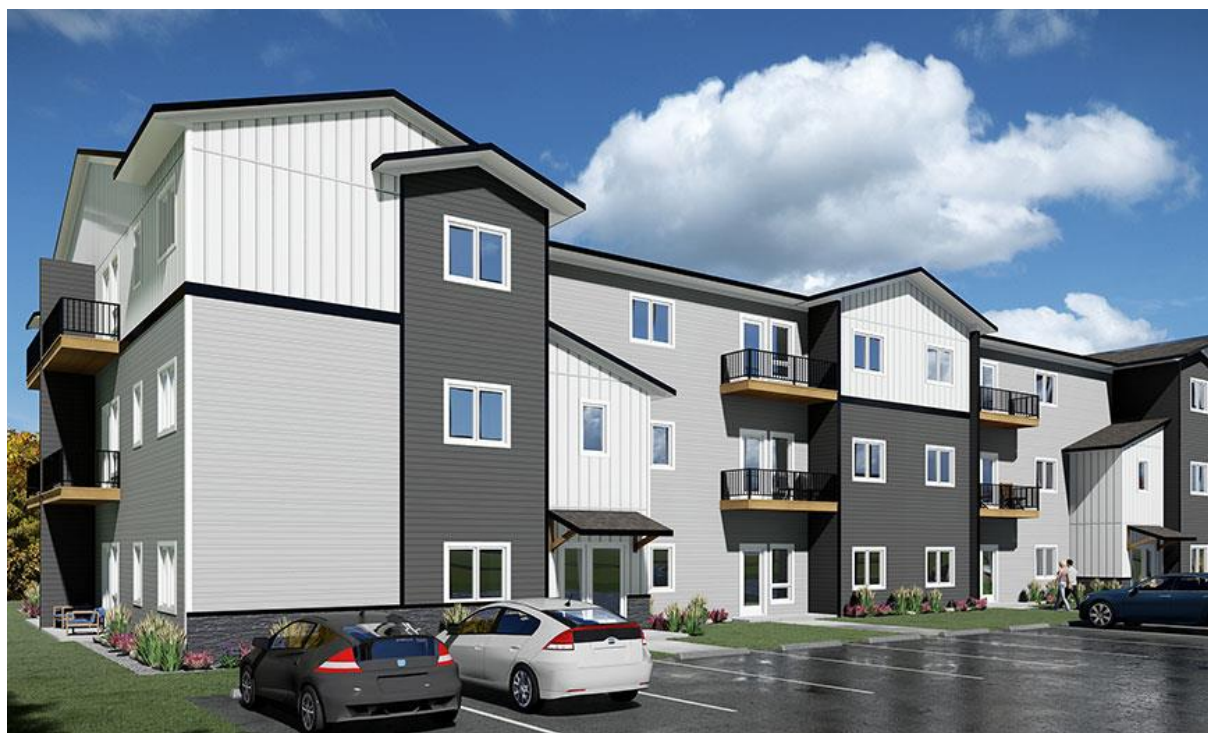
Figure 10: Greensmith Builders multi-family building STCBT pilot test – exterior
