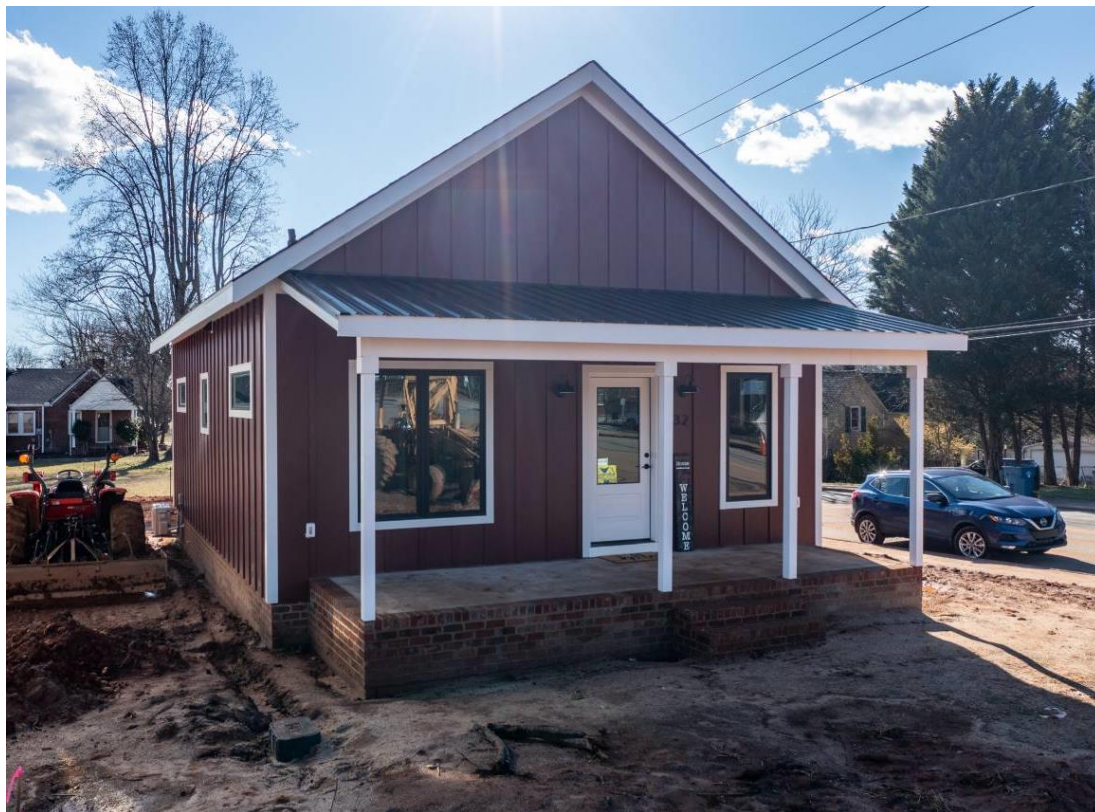
Figure 8: Howard Building Science single-family production home STCBT pilot test: Exterior
